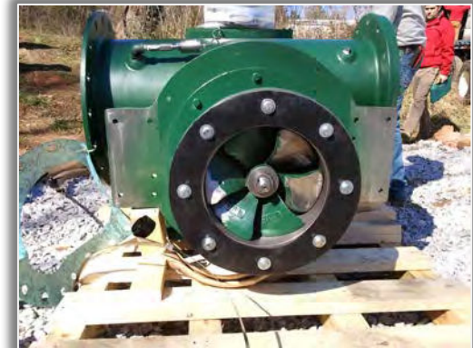
The turbine and runner was staged for placement on the platform.
