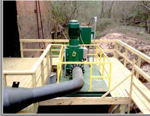
The decking and platform comply with OSHA and local regulations.
