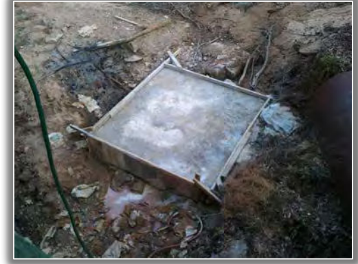
The 10' x 18' x 10" pad was required to support this entire system.
