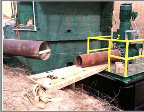
The penstock connections are typically performed last.
