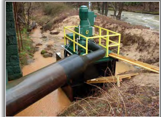
The turbine is complete and ready for the tour decking.
