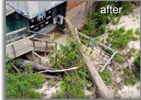
For 3 hours, the VFH was 18ft. under water but operational within 48 hrs.
