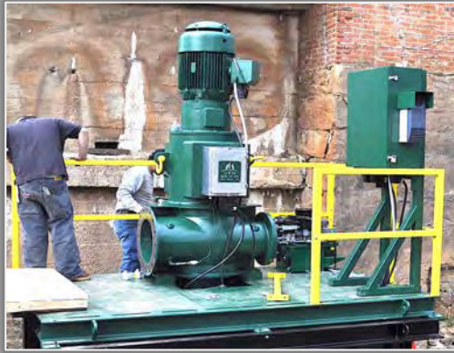
Once the platform has been placed, VFH assembly is 2 days.
